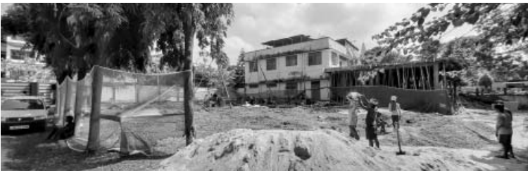
Construction work for the “Mission Home” started
